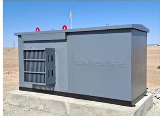
Figure 5: The first early works mini sub-station installed on site.
