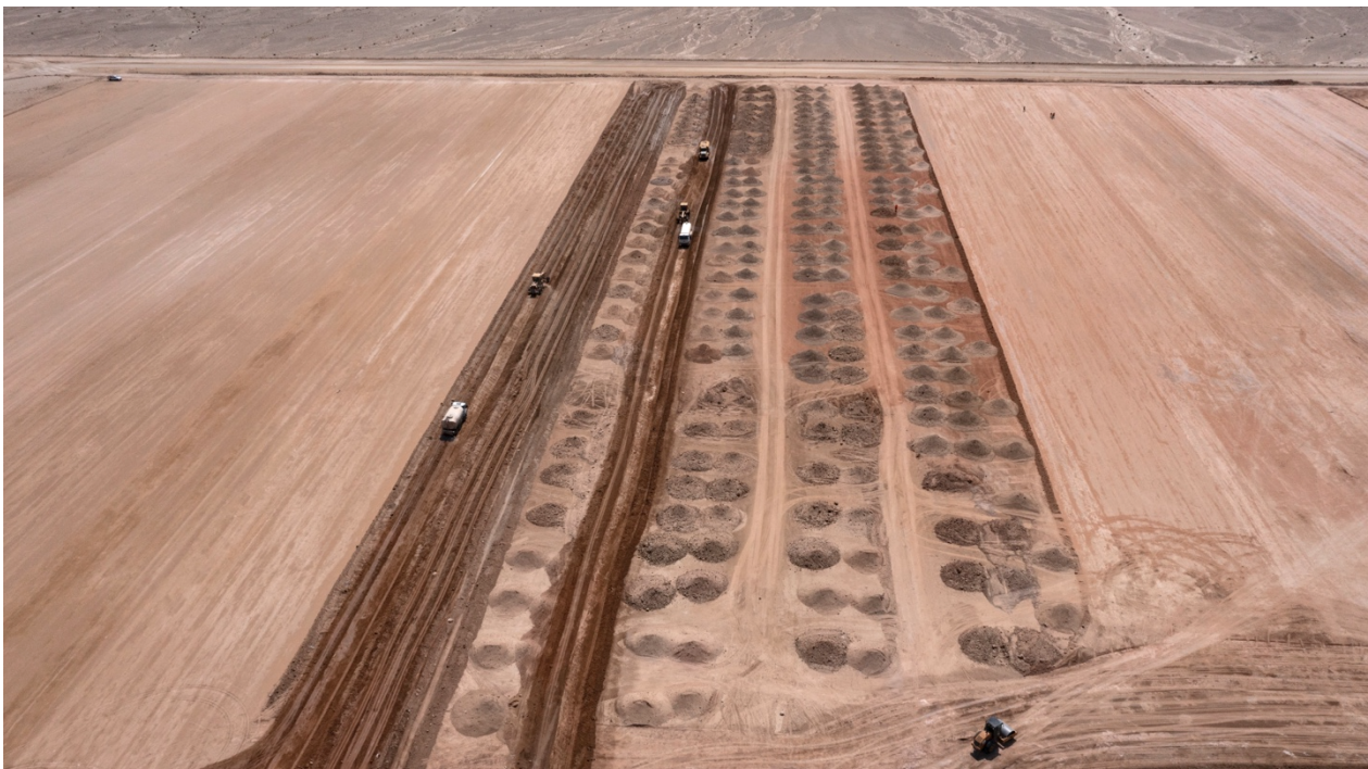
Figure 1: Heap leach earthworks continue to advance strongly.
